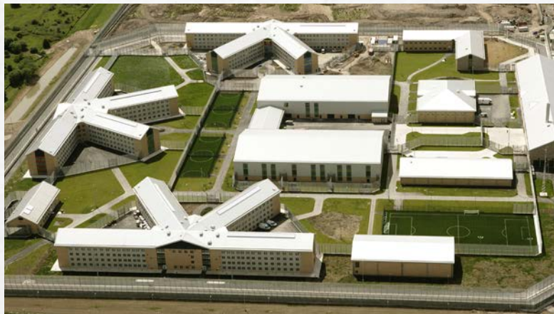
HM Prison Berwyn, Wales (Quelle: J. Williams, Precast Concrete Structures Ltd (PCS))
